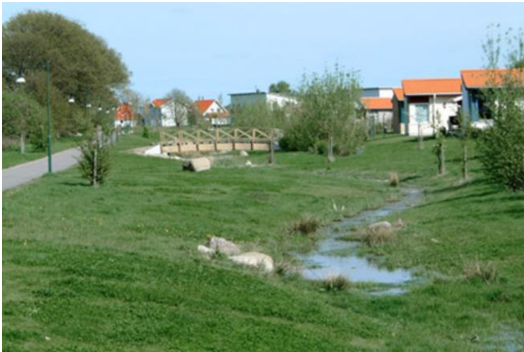
Figur 6.2.3 Utformning meandrande diken, princip (foto NSVA)
